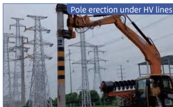
Reconstruction and construction under complex lines
